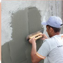
G-FIX-RAPIDPOWER mortar is applied to entire surface with circular motions by a 10 mm notched trowel. To get high adhesion strength for coating materials heavier than 30 kg/m<sup>2</sup>, G-FIX-RAPIDPOWER mortar should be applied on the backside of coating material too by a notched trowel before fixing. As G-FIX-RAPIDPOWER is a fast setting adhesive, it is necessary to work by dividing the application surface into small areas.
