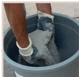
25 kg G-FIX-BLOCK laying adhesive is added on 6 liters of clean water by sprinkling.
