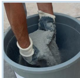
25 kg G-FIX-POWER tile adhesive is added on 7,5 liters of clean water by sprinkling.
