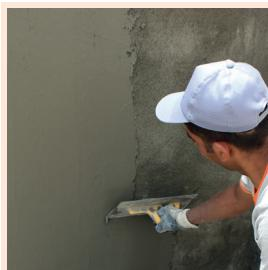
G-PLAST-800 mortar is applied to entire surface uniformly with a maximum thickness of 5 mm by a steel trowel.
