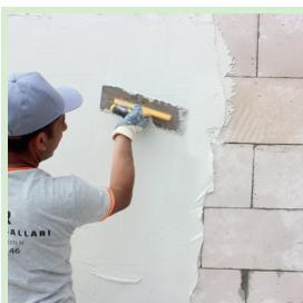
W-PLAST-1200 mortar is applied to entire surface uniformly with a maximum thickness of 1,5 cm by a steel trowel.
