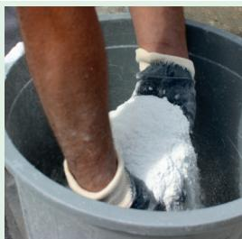
10 kg W-PLAST-THERM plaster is added on 11 liters of clean water by sprinkling.
