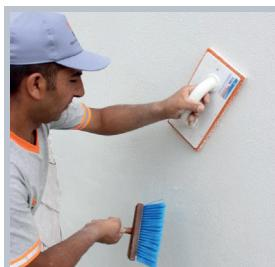
When plaster surface starts getting dry, it is smoothed with water using finishing trowel.
