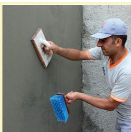
When plaster surface starts getting dry, it is corrected with water using finishing trowel.
