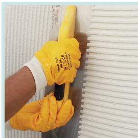
W-FIX-GRANIFLEX mortar is applied to entire surface with circular motions by a 10 mm notched trowel.
