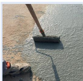
After taping is finished, HYDRO-G10 mortar is applied as 1 mm on the surface in one direction brush strokes as 1st layer by a roller or brush.
