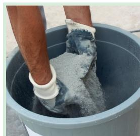
35 kg G-PLAST-1200 hand plaster is added on 7,5 liters of clean water by sprinkling.
