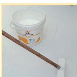
After approx. 6 hours from 1st layer application (when surface is completely dry), HYDRO-LP is applied on the entire surface in reverse direction brush strokes with a 1 mm thickness as 2nd layer.
