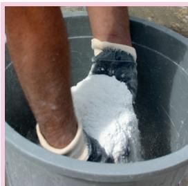
20 kg C-FUGA-ST joint filler mortar is added on 6,5 liters of clean water by sprinkling.
