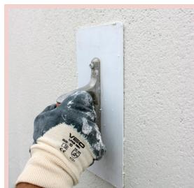
Approximately 10 min. after application, surface is decorated with vertical, horizontal or circular motions using a plastic trowel.
