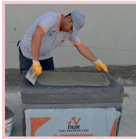
G-FIX-MANTO mortar is applied uniformly to entire backside surface of the thermal insulation board by leaving 5 mm from the edges of board with circular motions using minimum 10 mm notched trowel.
