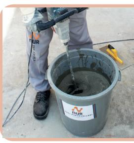
Mortar is blended by a low speed mixer to ensure that there are no lumps in it.
