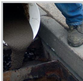
G-GROUT-RAPID mortar should be poured on one side of the mold.
