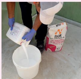
20 kg HYDRO-W10 powder comp. is added on 10 kg HYDRO-UV10 liquid component by sprinkling.
