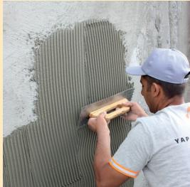
G-FIX-FLEX mortar is applied to entire surface with circular motions by a 8 mm notched trowel.
