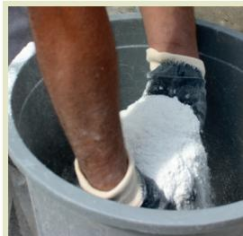
25 kg W-FIX-EXTRA tile adhesive is added on 6,5 liters of clean water by sprinkling.
