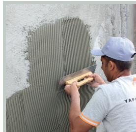
G-FIX-EXTRA mortar is applied to entire surface with circular motions by a 8 mm notched trowel.
