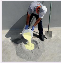
**Usage With Dry Readymix Cementious Mortars:** Dry readymix product is added on ADD-M1/water mixture prepared with a ratio 1:10. Drymix and ADD-M1/water mixture ratio should be in accordance with the ratio given in "PRODUCT INFORMATION FORM" of the drymix product. Mortar is blended by a low speed mixer and applied thorough it's "PRODUCT INFORMATION FORM".
