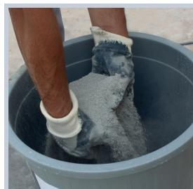
25 kg G-FIX-ECO tile adhesive is added on 6 liters of clean water by sprinkling.
