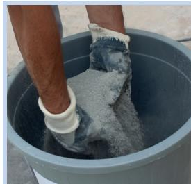
25 kg G-REPAIR-1200 coarse repair mortar is added on 6 liters of clean water by sprinkling.
