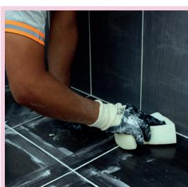
Depending on the ambient temperature approximately 20 minutes after the application, joints and coating materials are cleaned using a dry and clean sponge.
