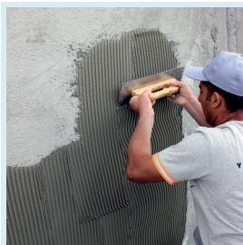
G-FIX-POOL mortar is applied to entire surface with circular motions by a 10 mm notched trowel.
