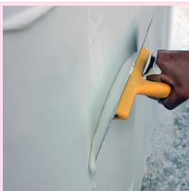
Finally surface smoothing is made with water and a steel trowel for a few times before surface gets completely dry.
