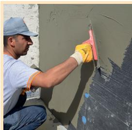
G-PLAST-MANTO mortar is applied uniformly to entire surface as 2 mm thickness as the 1.st layer by a steel trowel.
