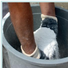
25 kg W-FIX-GRANIFLEX tile adhesive is added on 7,5 liters of clean water by sprinkling.
