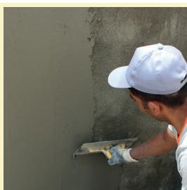
G-PLAST-POWER mortar is applied to entire surface uniformly with a maximum thickness of 5 mm by a steel trowel.
