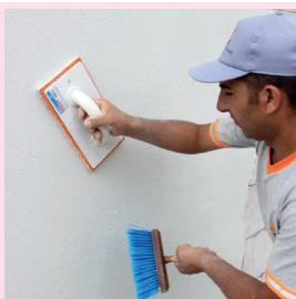
When plaster surface starts getting dry, it is corrected with water and finishing trowel. If 2nd layer application will be done, 1st layer shouldn't be smoothed.
