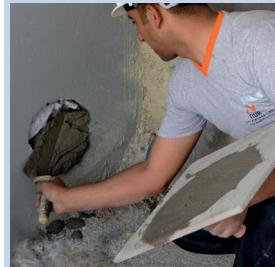
G-REPAIR-1200 mortar is filled with a trowel by applying pressure into the cracked area at a maximum depth of 40 mm.
