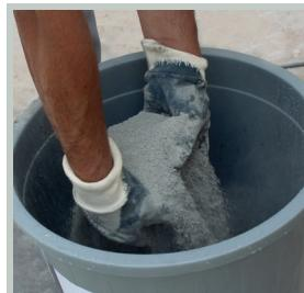
25 kg G-FIX-EXTRA tile adhesive is added on 6,5 liters of clean water by sprinkling.
