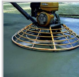
When surface is hard enough to walk on it, surface is smoothed by a mechanical floating trowel at high speed for a second time.
