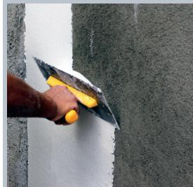
W-PLAST-POWER mortar is applied to entire surface uniformly with a maximum thickness of 5 mm by a steel trowel.
