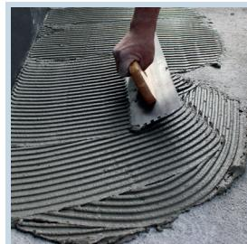
G-FIX-POWER mortar is applied to entire surface with circular motions by a 10 mm notched trowel.
