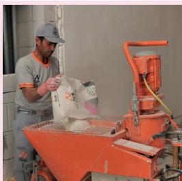
35 kg W-PLAST-MACHINE machine plaster is poured into the hopper of the plaster spraying machine. Water-plaster ratio of the machine should be fixed as 8 liters of clean water for 35 kg W-PLAST-MACHINE. Hopper of the machine shouldn't be empty during the application.
