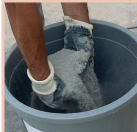
25 kg G-FIX-DECO adhesive is added on 6 liters of clean water by sprinkling.
