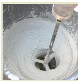
Mortar is blended by a low speed mixer or by a trowel to ensure that there are no lumps in it.
