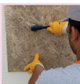
Coating material is fixed to the surface by gently tapping with a rubber mallet.
