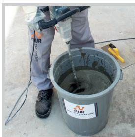
Mortar is blended by a low speed mixer or by a trowel to ensure that there are no lumps in it.
