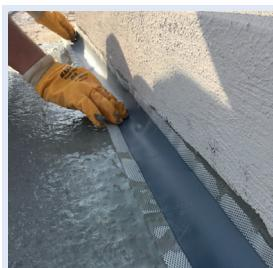
Prepared HYDRO-G10 mortar is applied to the corners and joints with a small brush as a thin layer.
