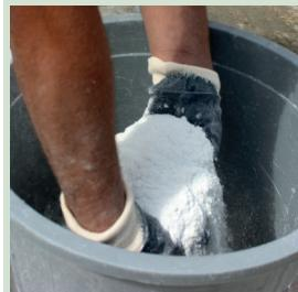
20 kg C-FUGA-FLEX joint filler mortar is added on 6,5 liters of clean water by sprinkling.
