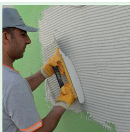
W-PLAST-THERM mortar is applied to entire surface uniformly with an 1,5 cm application thickness by a 15 mm notched trowel.
