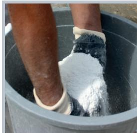
35 kg W-PLAST-POWER fine hand plaster is added on 8 liters of clean water by sprinkling.
