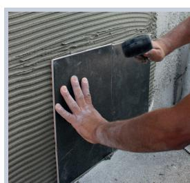
Coating material is fixed to the surface by gently tapping with a rubber mallet.
