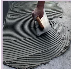
G-FIX-POWERFLEX mortar is applied to entire surface with circular motions by a 10 mm notched trowel.
