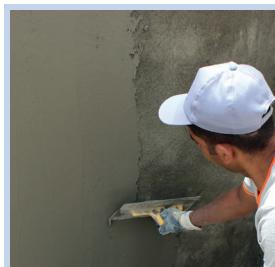
After crack is fully filled with mortar, the application surface is smoothed with G-REPAIR-1200 mortar by using trowel.
