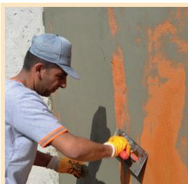
When plaster surface starts getting dry, G-PLAST-MANTO mortar is applied to entire surface as 1 mm thickness as the 2.nd layer by a trowel.
