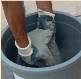
25 kg G-FIX-FLEX tile adhesive is added on 7,5 liters of clean water by sprinkling.
