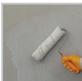
CURE-AR or CURE-HR concrete curing materials should be applied on all exposed surfaces after mortar surface starts drying.
