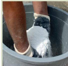
20 kg C-FUGA-SILFLEX joint filler mortar is added on 6,25 liters of clean water by sprinkling.
