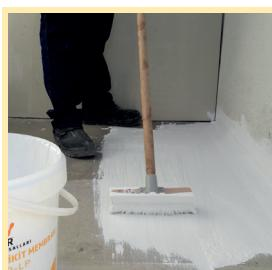
After taping is finished, HYDRO-LP is applied on the entire surface in one direction strokes with a 1 mm thickness as 1st layer by a roller or brush.
