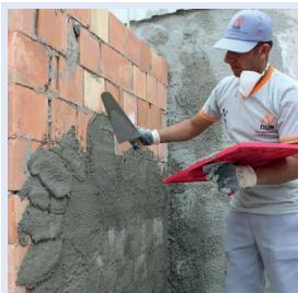
G-PLAST-2000 mortar is applied to entire surface uniformly with a maximum thickness of 3 cm by a steel trowel.
