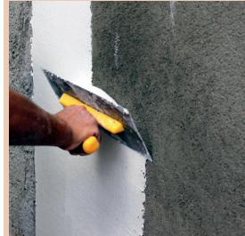
W-PLAST-800 mortar is applied to entire surface uniformly with a maximum thickness of 5 mm by a steel trowel.
