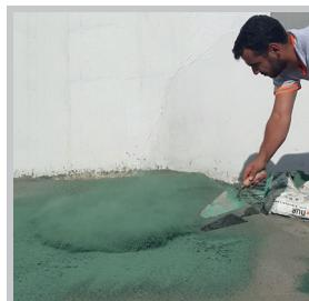
25 kg C-FLOOR-HARDENER surface hardener is ready for use, it is applied as powder. No mortar preparation is required. C-FLOOR-HARDENER surface hardener is sprinkled uniformly and evenly on the entire concrete surface as 5 kg/m<sup>2</sup> for grey color and as 8 kg/m<sup>2</sup> for other colors.
