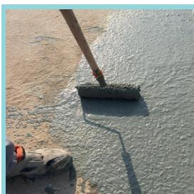
After taping is finished, HYDRO-G5 mortar is applied as 1 mm on the surface in one direction brush strokes as 1st layer by a roller or brush.
