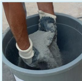
25 kg G-FIX-POOL tile adhesive is added on 7,5 liters of clean water by sprinkling.
