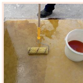
CURE-HR is ready to use, should be shaken before use. If it will be applied with roller, it is poured into a clean and wide bucket.
