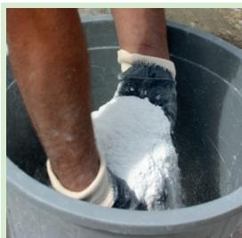
35 kg W-PLAST-1200 hand plaster is added on 7,5 liters of clean water by sprinkling.
