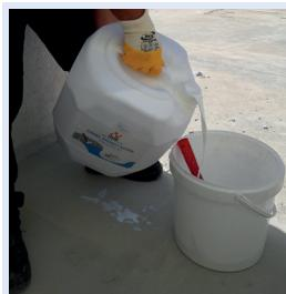
PRIMER-ST primer for general purpose is ready for use. Primer is poured into a clean and wide bucket.
