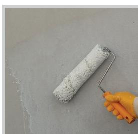
CURE-AR or CURE-HR concrete curing materials should be applied on all exposed surfaces after mortar surface starts drying.
