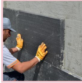
Thermal insulation board is placed without fuga gaps and fixed to the surface by gently tapping with a rubber mallet.
