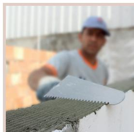
G-FIX-BLOCK mortar is applied to entire fixing surface uniformly and evenly by a minimum 8 mm notched trowel.
