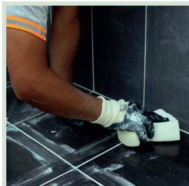
Depending on the ambient temperature approximately 20 minutes after the application, joints and coating materials are cleaned a dry and clean sponge.
