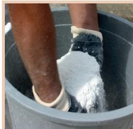
35 kg W-PLAST-800 fine hand plaster is added on 8 liters of clean water by sprinkling.
