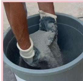
25 kg G-FIX-MANTO thermal insulation board adhesive is added on 6 liters of clean water by sprinkling.
