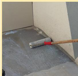
PRIMER-ST primer should be used at least 1 hour before the application to reduce water absorption of the surface and to provide better adhesion.
