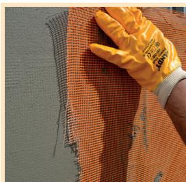
THERMMESH-A1 glass-fiber mesh should be placed by stretching while 1st layer mortar surface is still fresh. Mesh should be embeded on plaster as gently pressing from bottom to top by a trowel.
