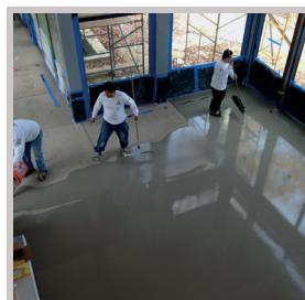
G-FLOOR-SELF mortar is poured on surface, it can be helped to spread the mortar with a trowel.
