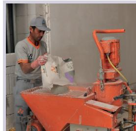
35 kg G-PLAST-MACHINE machine plaster is poured into the hopper of the plaster spraying machine. Water-plaster ratio of the machine should be fixed as 8 liters of clean water for 35 kg G-PLAST-MACHINE. Hopper of the machine shouldn't be empty during the application.
