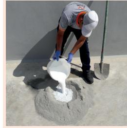
**Application as Mortar Additive:** A mixing solution is prepared by mixing ADD-LATEX with clean water at a ratio between 1:3 to 1:4.
