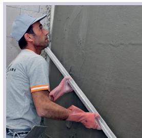
After spraying is completed, fresh plaster surface is smoothed by a template.
