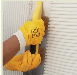
W-FIX-EXTRA mortar is applied to entire surface with circular motions by a 8 mm notched trowel.
