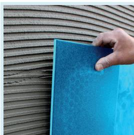
Coating material is placed on surface by setting fuga gaps.
