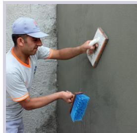
When plaster surface starts getting dry, it is corrected with water and finishing trowel. If 2nd layer application will be done, 1st layer shouldn't be smoothed.
