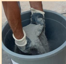
25 kg G-PLAST-MANTO thermal insulation board plaster is added on 6 liters of clean water by sprinkling.
