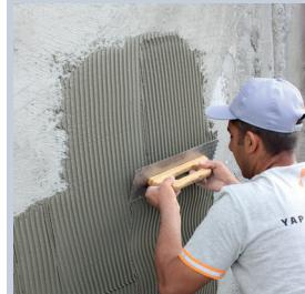
G-FIX-ECO mortar is applied to entire surface with circular motions by a 6 mm notched trowel.
