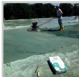
Hardener is matured until it absorb water from concrete surface and get wet. Surface is smoothed by using a mechanical floating trowel.
