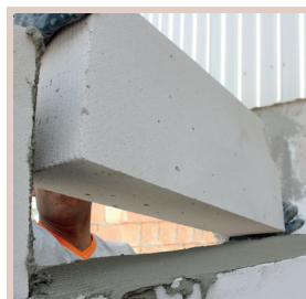
After the mortar application, laying material is placed through plumb line of the wall by setting fuga gaps.
