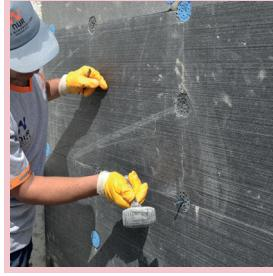
Minimum 24 hours after fixing of thermal insulation boards, 6 holes are drilled for each 1 m<sup>2</sup> by a drill with a suitable width, especially at the junctions of the plates. THERMFIX-10 anchors are inserted into these holes and fixed by tapping with a rubber mallet.
