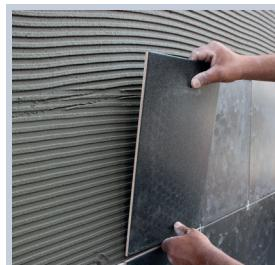
Coating material is placed on surface by setting fuga gaps.
