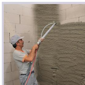
G-PLAST-MACHINE machine plaster is sprayed to the surface with spraying machine. Applications thickness should be max. 1,5 cm in a single layer. In case application thickness exceeds 1,5 cm, 2.nd layer application should be done after 1 day from 1st layer application.
