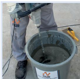
Mortar is blended by a low speed mixer to ensure that there are no lumps in it.
