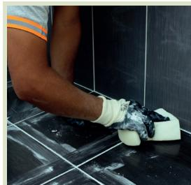
Depending on the ambient temperature approximately 20 minutes after the application, joints and coating materials are cleaned using a dry and clean sponge.
