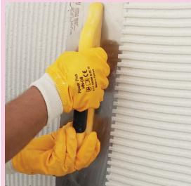
W-FIX-GRANITE mortar is applied to entire surface with circular motions by a 10 mm notched trowel.
