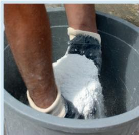
20 kg C-FUGA-POOL joint filler mortar is added on 6,25 liters of clean water by sprinkling.
