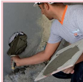
G-REPAIR-800 mortar is filled with a trowel by applying pressure into the cracked area at a maximum depth of 20 mm.
