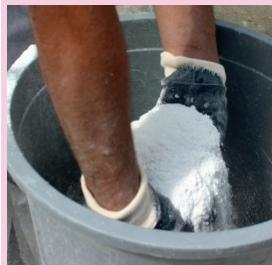
25 kg W-FIX-GRANITE tile adhesive is added on 7,5 liters of clean water by sprinkling.
