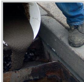
G-GROUT-ST mortar should be poured slowly on one side of the mold.
