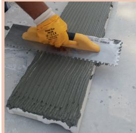
G-FIX-DECO mortar is applied uniformly to entire backside surface of foam element by leaving 5 mm from the edges of board with circular motions using minimum 8 mm notched trowel.
