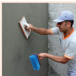
When plaster surface starts getting dry, it is corrected with water and finishing trowel.
