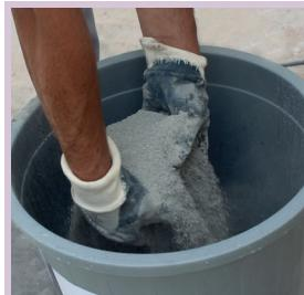
25 kg G-FIX-POWERFLEX tile adhesive is added on 7,5 liters of clean water by sprinkling.
