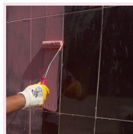
PRIMER-TILE adhesion enhancing primer is ready for use. Should be mixed until it becomes homogenous before starting to use.
