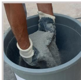
25 kg G-FLOOR-SELF floor levelling mortar is added on 6 liters of clean water by sprinkling.
