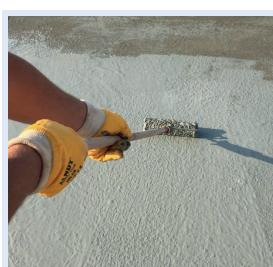
After 6 hours from 1st layer application (before surface completely dry), prepared HYDRO-G10 mortar is applied on the entire surface in reverse direction brush strokes with a 1 mm thickness as 2nd layer.
