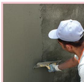
After crack is fully filled with mortar, the application surface is smoothed with G-REPAIR-800 mortar by using trowel.
