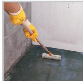
When C-FLOOR-HARDENER surface hardener application is complete and the surface begins to lose its free water (when it becomes dull), CURE-AR or CURE-HR concrete curing material must be applied to the surface to prevent stress cracks and dust formation due to sudden water losses. CURE-AR or CURE-HR should be shaked before using. It is applied uniformly and evenly to entire surface by a roller, brush or a spraying machine.
