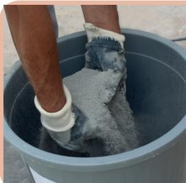
Adhesive/water ratio is determined as 7,5 liters of clean water for 25 kg G-FIX-RAPIDPOWER. As G-FIX-RAPIDPOWER is a rapid setting adhesive, it should be mixed in small amounts and should be applied without any delay after mixing.
