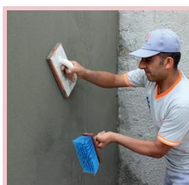
If neeed, surface is smoothed with water by using finishing trowel when mortar surface starts getting dry.
