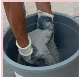
25 kg G-REPAIR-800 fine repair mortar is added on 6 liters of clean water by sprinkling.
