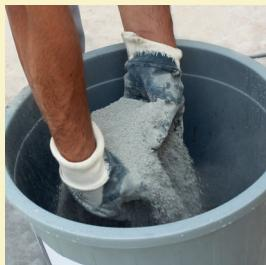
35 kg G-PLAST-POWER fine hand plaster is added on 8 liters of clean water by sprinkling.
