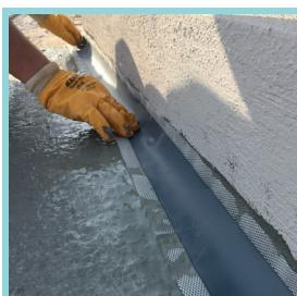
Prepared HYDRO-G5 mortar is applied to the corners and joints with a small brush as a thin layer.
