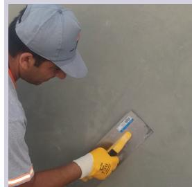
Final smoothing is made with water and a steel trowel for a few times before surface gets completely dry.
