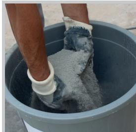
25 kg G-GROUT-ST repair mortar is added on 3,5 liters of clean water by sprinkling.
