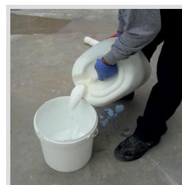
CURE-AR is ready to use, should be shaken before use. If it will be applied with roler, it is poured into a clean and wide bucket.
