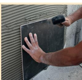
Coating material is fixed to the surface by gently tapping with a rubber mallet.
