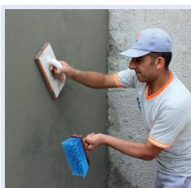
In case application thickness exceeds 3 cm, 2nd layer application should be done after 1 day from 1st layer.
