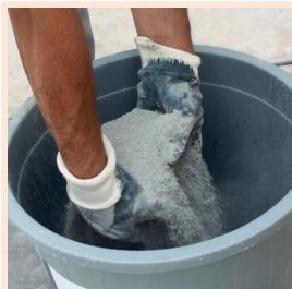
35 kg G-PLAST-800 fine plaster is added on 8 liters of clean water by sprinkling.
