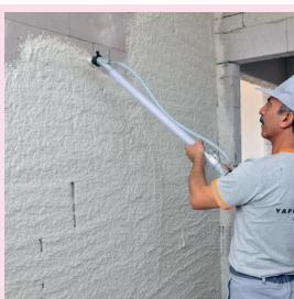
W-PLAST-MACHINE machine plaster is sprayed to the surface with spraying machine. Applications thickness should be max. 1,5 cm in a single layer. In case application thickness exceeds 2 cm, 2nd layer application should be done after 1 day from 1st layer application.
