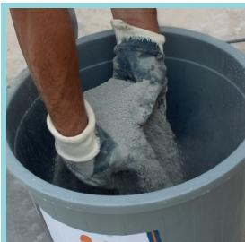
20 kg HYDRO-G5 powder component is added on 5 kg HYDRO-L5 liquid component by sprinkling.
