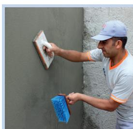
If neeed, surface is smoothed with water by using finishing trowel when mortar surface starts getting dry.
