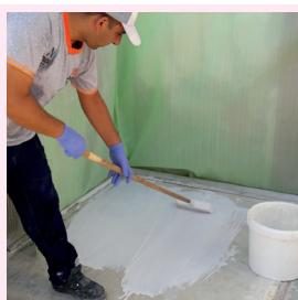
After taping is finished, HYDRO-W10 mortar is applied as 1 mm on the surface in one direction brush strokes as 1st layer by a roller or brush.
