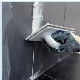
C-FUGA-POOL mortar is filled in joints between coating materials by applying pressure with a rubber trowel.
