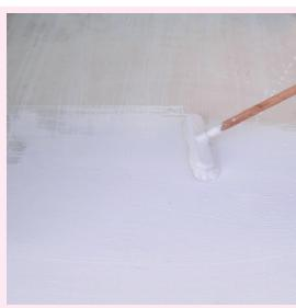
After 6 hours from 1st layer application (before surface completely dry), prepared HYDRO-W10 mortar is applied on the entire surface in reverse direction brush strokes with a 1 mm thickness as 2nd layer.
