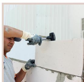
Laying material is fixed to the surface by gently tapping with a rubber mallet.
