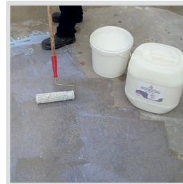
**For Concrete Applications:** Cure application should be start when freshly poured concrete surface starts tarnishing (when free water disappears). For concrete application with molds, cure should be applied immediately after removal of molds.
