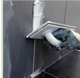
C-FUGA-SILFLEX mortar is filled in joints between coating materials by applying pressure with a rubber trowel.
