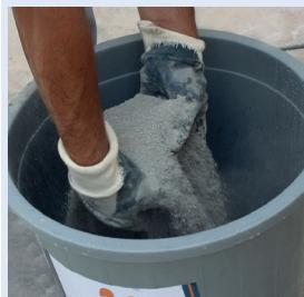
20 kg HYDRO-G10 powder component is added on 10 kg HYDRO-L10 liquid component by sprinkling.
