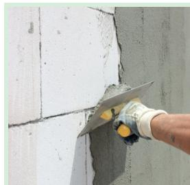
G-PLAST-1200 mortar is applied to entire surface uniformly with a maximum thickness of 1,5 cm by a steel trowel.
