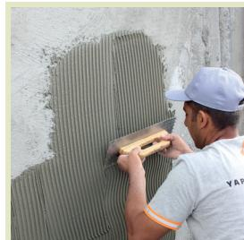
G-FIX-ST mortar is applied to entire surface with circular motions by a 6 mm notched trowel.
