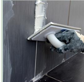
C-FUGA-FLEX mortar is filled in joints between coating materials by applying pressure with a rubber trowel.
