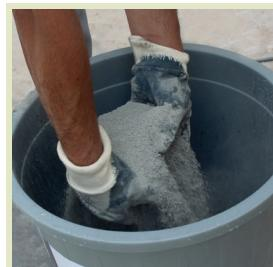
25 kg G-FIX-ST tile adhesive is added on 6,25 liters of clean water by sprinkling.
