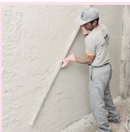
After spraying is completed, fresh plaster surface is smoothed by a template.
