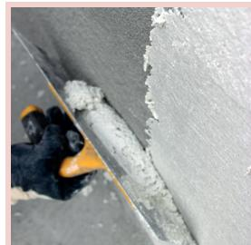
W-PLAST-DECO is applied to entire surface uniformly with a thickness of 2 mm by a steel trowel as the finishing layer.
