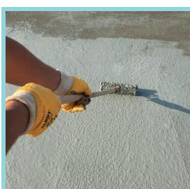
After 6 hours from 1st layer application (before surface completely dry), prepared HYDRO-G5 mortar is applied on the entire surface in reverse direction brush strokes with a 1 mm thickness as 2nd layer.
