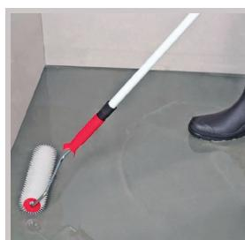
Air bubbles on surface are removed by using a spiked roller for minimum 3 times.
