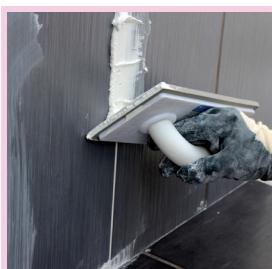
C-FUGA-ST mortar is filled in joints between coating materials by applying pressure with a rubber trowel.
