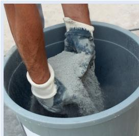
35 kg G-PLAST-2000 coarse hand plaster is added on 5,5 liters of clean water by sprinkling.
