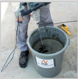
Mortar is blended by a low speed mixer or by a trowel to ensure that there are no lumps in it. Mortar should be applied without delay.
