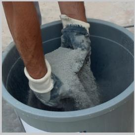
25 kg G-GROUT-RAPID repair mortar is added on 4,0 liters of clean water by sprinkling.
