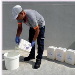
**Usage With Dry Readymix Cementitious Mortars:** Dry readymix product is added on ADD-M1/water mixture prepared with a ratio 1:10. Drymix and ADD-M1/water mixture ratio should be in accordance with the ratio given in "PRODUCT INFORMATION FORM" of the drymix product. Mortar is blended by a low speed mixer and applied through it's "PRODUCT INFORMATION FORM".
