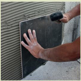
Coating material is fixed to the surface by gently tapping with a rubber mallet. Joint filler application should be done at least 24 hours after fixing.
