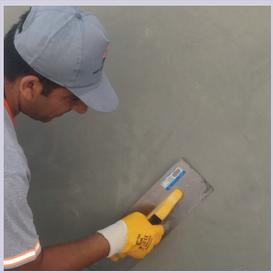
Final smoothing is made with water and a steel trowel for a few times before surface gets completely dry. After setting time is completed, surface becomes ready for other applications on it.
