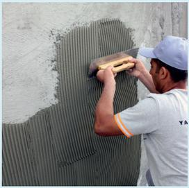
G-FIX-POOL mortar is applied to entire surface with circular motions by a 10 mm notched trowel. To get high adhesion strength for the coating materials heavier than 30 kg/m<sup>2</sup>, G-FIX-POOL mortar should be applied on backside of coating material too by a notched trowel before fixing.
