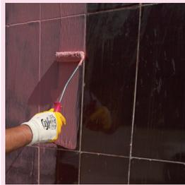
PRIMER-TILE adherence enhancing primer is ready for use. Should be mixed until it becomes homogenous before starting to use.
