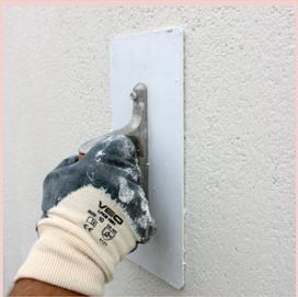
Approximately 10 min. after application, surface is decorated with vertical, horizontal or circular motions using a plastic trowel.
