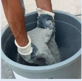
35 kg G-PLAST-2000 coarse hand plaster is added on 5,5 liters of clean water by sprinkling.
