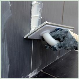
C-FUGA-FLEX mortar is filled in joints between coating materials by applying pressure with a rubber trowel. Excess mortar on the surface is removed by rubber trowel.
