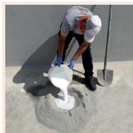
**Application as Primer:** A mixing solution is prepared by mixing ADD-LATEX with clean water at a ratio 1:1. Prepared mixing solution is added to cement/aggregate mixture with a ratio of 1:1. It is blended by a low speed mixer to get a consistent primer mortar.
