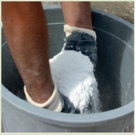
20 kg C-FUGA-SILFLEX joint filler mortar is added on 6,25 liters of clean water by sprinkling.
