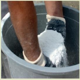
25 kg W-FIX-EXTRA tile adhesive is added on 6,5 liters of clean water by sprinkling.
