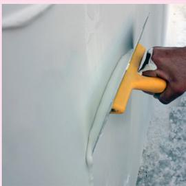
Finally surface smoothing is made with water and a steel trowel for a few times before surface gets completely dry. After drying time is completed, surface becomes ready for other applications on it.
