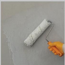
CURE-AR or CURE-HR concrete curing materials should be applied on all exposed surfaces after mortar surface starts drying. Molds should be taken off after G-GROUT-RAPID mortar is fully cured. After drying time is completed, surface becomes ready to use.
