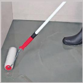
Air bubbles on surface are removed by using a spiked roller for minimum 3 times. Spiked shoes should be worn to avoid footprints on the mortar during the application.
