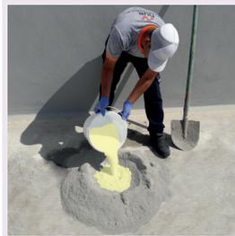
**Usage With Screed Prepared By Mixing Cement & Aggregate:** After primer application, screed application is done in 2 layers; 1st adhesion layer, 2nd main floor layer. 1st adhesion layer should be minimum 10 mm thickness and leveled by steel trowel. 2nd main floor layer should be minimum 30 mm thickness and leveled by a wooden trowel after tamping.
