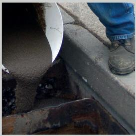
G-GROUT-ST mortar should be poured slowly on one side of the mold. Air bubbles forming should be avoided while pouring the mortar. Casting on both sides of the mold should never be done. G-GROUT-ST mortar should be applied as minimum 10 mm and maximum 70 mm thickness.
