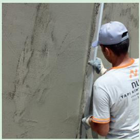
After the application, fresh mortar surface is smoothed by a template. In case application thickness exceeds 1,5 cm, 2nd layer application should be done after 1 day from 1st layer.
