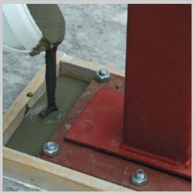
It is recommended to consume the mortar within 15 minutes for maximum performance. Since air bubbles will reduce adhesion and compressive strength, it should be ensured that no air bubbles remain during casting.
