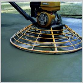
When surface is hard enough to walk on it, surface is smoothed by a mechanical floating trowel at high speed for a second time.
