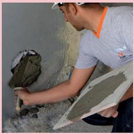
G-REPAIR-800 mortar is filled with a trowel by applying pressure into the cracked area at a maximum depth of 20 mm. If crack is deeper than 20 mm, 2nd layer application should be done 1 day after 1st layer application.
