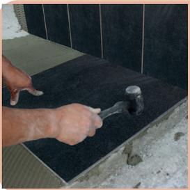
Coating material is fixed to the surface by gently tapping with a rubber mallet. It is recommended that the application tools be cleaned immediately after the application. Joint filler application should be done at least 6 hours after fixing.
