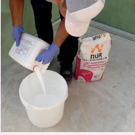
20 kg HYDRO-W10 powder comp. is added on 10 kg HYDRO-UV10 liquid component by sprinkling.
