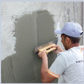
G-FIX-ECO mortar is applied to entire surface with circular motions by a 6 mm notched trowel. To get high adhesion strength for the coating materials heavier than 7 kg/m<sup>2</sup>, G-FIX-ECO mortar should be applied on backside of coating material too by a notched trowel before fixing.
