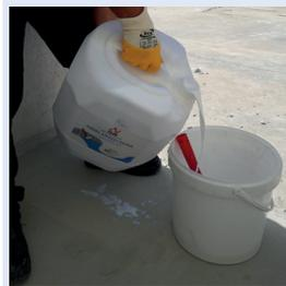
PRIMER-ST primer for general purpose is ready for use. Primer is poured into a clean and wide bucket. PRIMER-ST primer for general purpose is applied uniformly to entire surface with a roller or brush as a thin layer.
