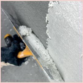
W-PLAST-DECO is applied to entire surface uniformly with a thickness of 2 mm by a steel trowel as the finishing layer. Not to get any difference pattern on the surface, same water-plaster ratio should be used for each mixing.
