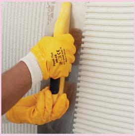
W-FIX-GRANITE mortar is applied to entire surface with circular motions by a 10 mm notched trowel. To get high adhesion strength for the coating materials heavier than 30 kg/m<sup>2</sup>, W-FIX-GRANITE mortar should be applied on backside of coating material too by a notched trowel before fixing.
