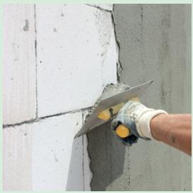
G-PLAST-1200 mortar is applied to entire surface uniformly with a maximum thickness of 1,5 cm by a steel trowel.
