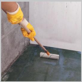
When C-FLOOR-HARDENER surface hardener application is complete and the surface begins to lose its free water (when it becomes dull), CURE-AR or CURE-HR concrete curing material must be applied to the surface to prevent stress cracks and dust formation due to sudden water losses. CURE-AR or CURE-HR should be shaken before using. It is applied uniformly and evenly to entire surface by a roller, brush or a spraying machine.
