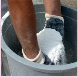
25 kg W-FIX-GRANITE tile adhesive is added on 7,5 liters of clean water by sprinkling.
