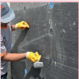
Minimum 24 hours after fixing of thermal insulation boards, 6 holes are drilled for each 1 m<sup>2</sup> by a drill with a suitable width, especially at the junctions of the plates. THERMFIK-10 anchors are inserted into these holes and fixed by tapping with a rubber mallet. After anchor application is finished, board surface becomes ready for plaster application on it.
