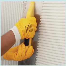
W-FIX-GRANIFLEX mortar is applied to entire surface with circular motions by a 10 mm notched trowel. To get high adhesion strength for the coating materials heavier than 30 kg/m<sup>2</sup>, W-FIX-GRANIFLEX mortar should be applied on backside of coating material too by a notched trowel before fixing.
