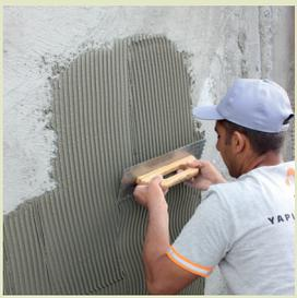
G-FIX-ST mortar is applied to entire surface with circular motions by a 6 mm notched trowel. To get high adhesion strength for the coating materials heavier than 10 kg/m<sup>2</sup>, G-FIX-ST mortar should be applied on backside of coating material too by a notched trowel before fixing.
