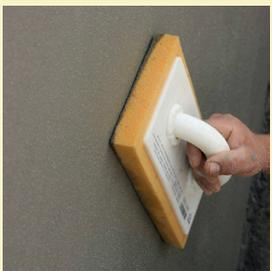
When plaster surface starts getting dry after the correction application, it is smoothed by using a damp sponge trowel. After drying time is completed, surface becomes ready for other applications on it.
