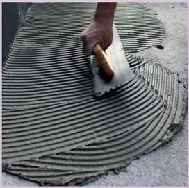
G-FIX-POWERFLEX mortar is applied to entire surface with circular motions by a 10 mm notched trowel. To get high adhesion strength for the coating materials heavier than 30 kg/m<sup>2</sup>, G-FIX-POWERFLEX mortar should be applied on backside of coating material too by a notched trowel before fixing.
