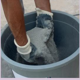
25 kg G-FIX-POWERFLEX tile adhesive is added on 7,5 liters of clean water by sprinkling.
