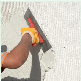
2nd layer application should be done after 1 day from 1st layer. W-PLAST-THERM mortar is applied to entire surface uniformly with an 1,5 cm application thickness by a steel trowel.
