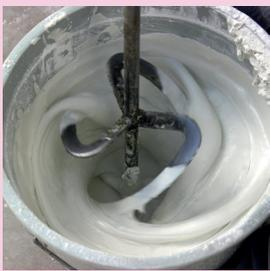
Mortar is blended by a low speed mixer or by a trowel to ensure that there are no lumps in it. Mortar is rested for 5 minutes to mature and mixed again before the application.
