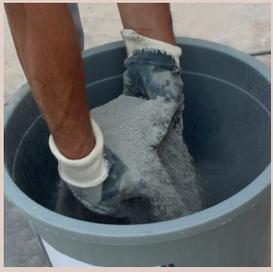
25 kg G-FIX-BLOCK laying adhesive is added on 6 liters of clean water by sprinkling.
