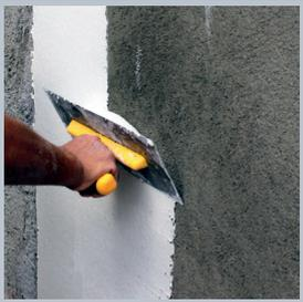
W-PLAST-POWER mortar is applied to entire surface uniformly with a maximum thickness of 5 mm by a steel trowel.
