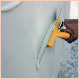
W-PLAST-FINISH mortar is applied to entire surface max. 2 mm thickness by a steel trowel.
