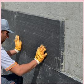
Thermal insulation board is placed without fuga gaps and fixed to the surface by gently tapping with a rubber mallet. After fixing of thermal insulation board, mortars overflowing from edges should be cleaned not to have gaps between boards.
