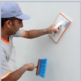
When plaster surface starts getting dry, it is smoothed with water using finishing trowel.
