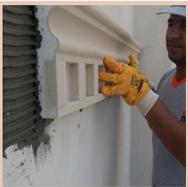
Decorative foam elements are placed on surface without leaving gaps. To get high adhesion strength, foam elements are fixed to the surface by gently tapping with a rubber mallet. After fixing of foam elements, mortars overflowing from the edges should be cleaned not to have gaps between the elements.
