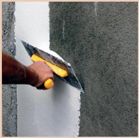
W-PLAST-800 mortar is applied to entire surface uniformly with a maximum thickness of 5 mm by a steel trowel.
