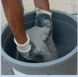
25 kg G-REPAIR-1200 coarse repair mortar is added on 6 liters of clean water by sprinkling.
