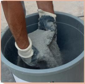
Adhesive/water ratio is determined as 7,5 liters of clean water for 25 kg G-FIX-RAPIDPOWER. As G-FIX-RAPIDPOWER is a rapid setting adhesive, it should be mixed in small amounts and should be applied without any delay after mixing. Tile adhesive is added on clean water by sprinkling.
