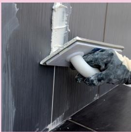
C-FUGA-ST mortar is filled in joints between coating materials by applying pressure with a rubber trowel. Excess mortar on the surface is removed by rubber trowel.
