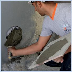
G-REPAIR-1200 mortar is filled with a trowel by applying pressure into the cracked area at a maximum depth of 40 mm. If crack is deeper than 40 mm, 2nd layer application should be done 1 day after 1st layer application.
