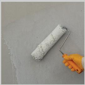
CURE-AR or CURE-HR concrete curing materials should be applied on all exposed surfaces after mortar surface starts drying. Molds should be taken off after G-GROUT-ST mortar is fully cured. After drying time is completed, surface becomes ready to use.
