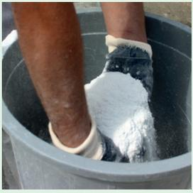
10 kg W-PLAST-THERM plaster is added on 11 liters of clean water by sprinkling. In order to obtain a homogeneous mortar, one full package should be used in each mixture and the water-dust ratio should be considered. Do not mix and use half package.
