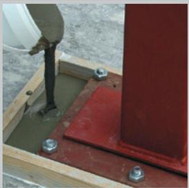
It is recommended to consume the mortar within 5-8 minutes for maximum performance. Since air bubbles will reduce adhesion and compressive strength, it should be ensured that no air bubbles remain during casting.
