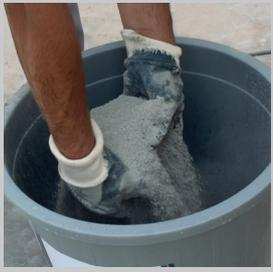
25 kg G-GROUT-ST repair mortar is added on 3,5 liters of clean water by sprinkling.
