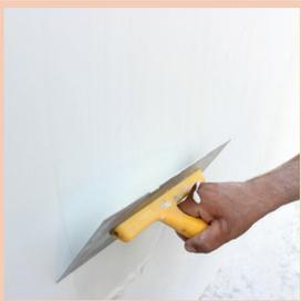
When plaster surface starts getting dry, it is smoothed with water and steel trowel for a few times. After drying time is completed, surface becomes ready for other applications on it.
