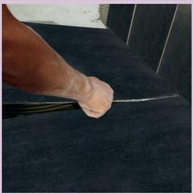
Coating material is placed on surface by setting fuga gaps. If a film layer formed on mortar surface, mortar should not be used. Mortar should be scraped off from surface and new mortar should be applied.
