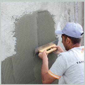
G-FIX-EXTRA mortar is applied to entire surface with circular motions by a 8 mm notched trowel. To get high adhesion strength for the coating materials heavier than 15 kg/m<sup>2</sup>, G-FIX-EXTRA mortar should be applied on backside of coating material too by a notched trowel before fixing.
