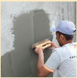
G-FIX-FLEX mortar is applied to entire surface with circular motions by a 8 mm notched trowel. To get high adhesion strength for the coating materials heavier than 15 kg/m<sup>2</sup>, G-FIX-FLEX mortar should be applied on backside of coating material too by a notched trowel before fixing.
