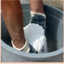
20 kg W-PLAST-FINISH satin finishing plaster is added on 7 liters of clean water by sprinkling.
