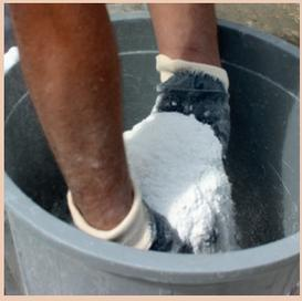
35 kg W-PLAST-800 fine hand plaster is added on 8 liters of clean water by sprinkling.
