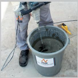
Mortar is blended by a low speed mixer or by a trowel to ensure that there are no lumps in it. Mortar should be applied without any delay. As the mortar sets very fast, the application tools should be cleaned immediately after the application.
