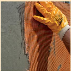
THERMMESH-A1 glass-fiber mesh should be placed by stretching while 1st layer mortar surface is still fresh. Mesh should be embedded on plaster as gently pressing from bottom to top by a trowel. It should be avoided from folding of glass-fiber mesh.
