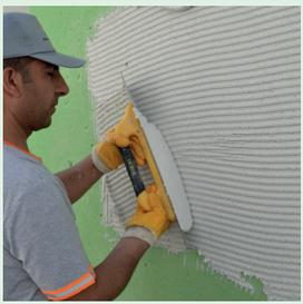
W-PLAST-THERM mortar is applied to entire surface uniformly with an 1,5 cm application thickness by a 15 mm notched trowel. When 1st layer surface is still fresh, plaster levelling bars is placed and fixed in accordance with the application thickness.
