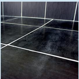
When joint filler surface starts getting dry, it is smoothed using a damp rag or sponge. Also coating material surface should be cleaned using a damp rag or sponge after joint filler surface starts drying. After the time required for opening to traffic is completed, surface becomes ready to use.
