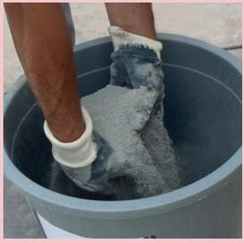
25 kg G-REPAIR-800 fine repair mortar is added on 6 liters of clean water by sprinkling.
