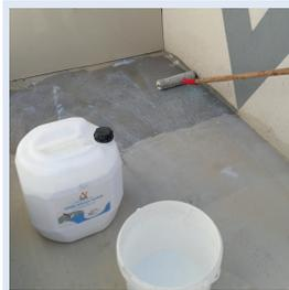
After drying time is completed, surface will be ready for the upper applications on it. Upper application should be done in 7 days after application, surface shouldn't be exposed to long term external effects.
