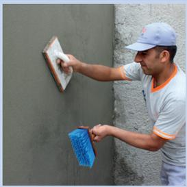
If needed, surface is smoothed with water by using finishing trowel when mortar surface starts getting dry. After drying time is completed, surface becomes ready for other applications on it.
