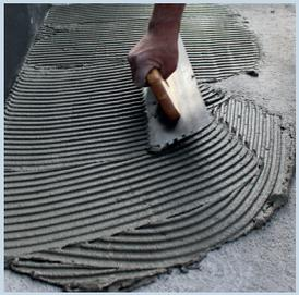
G-FIX-POWER mortar is applied to entire surface with circular motions by a 10 mm notched trowel. To get high adhesion strength for the coating materials heavier than 30 kg/m<sup>2</sup>, G-FIX-POWER mortar should be applied on backside of coating material too by a notched trowel before fixing.
