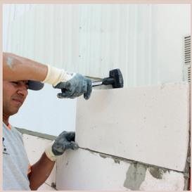
Laying material is fixed to the surface by gently tapping with a rubber mallet. After drying time is completed, wall becomes ready for other applications on it.
