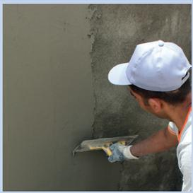
After crack is fully filled with mortar, the application surface is smoothed with G-REPAIR-1200 mortar by using trowel. If application area is wide and deep, glass-fiber mesh should be used to prevent formation of cracks on surface. Mesh is placed by stretching while mortar surface is still fresh. Mesh should be embedded on plaster as gently pressing by a trowel.
