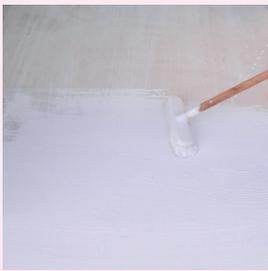
After 6 hours from 1st layer application (before surface completely dry), prepared HYDRO-W10 mortar is applied on the entire surface in reverse direction brush strokes with a 1 mm thickness as 2nd layer.
