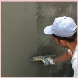
After crack is fully filled with mortar, the application surface is smoothed with G-REPAIR-800 mortar by using trowel. If application area is wide and deep, glass-fiber mesh should be used to prevent formation of cracks on surface. Mesh is placed by stretching while mortar surface is still fresh. Mesh should be embedded on plaster as gently pressing by a trowel.
