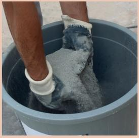
25 kg G-FIX-DECO adhesive is added on 6 liters of clean water by sprinkling.
