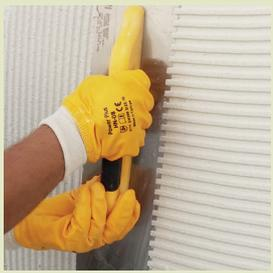
W-FIX-EXTRA mortar is applied to entire surface with circular motions by a 8 mm notched trowel. To get high adhesion strength for the coating materials heavier than 15 kg/m<sup>2</sup>, W-FIX-EXTRA mortar should be applied on backside of coating material too by a notched trowel before fixing.
