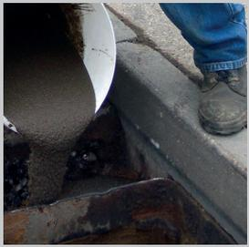
G-GROUT-RAPID mortar should be poured on one side of the mold. Air bubbles forming should be avoided while pouring the mortar. Casting on both sides of the mold should never be done. G-GROUT-RAPID mortar should be applied as minimum 10 mm and maximum 70 mm thickness.
