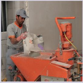
35 kg G-PLAST-MACHINE machine plaster is poured into the hopper of the plaster spraying machine. Water-plaster ratio of the machine should be fixed as 8 liters of clean water for 35 kg G-PLAST-MACHINE. Hopper of the machine shouldn't be empty during the application.
