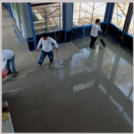
G-FLOOR-SELF mortar is poured on surface, it can be helped to spread the mortar with a trowel. Since the mortar can spread very well in the first 20 minutes, it should be applied during this time.
