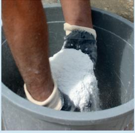
20 kg C-FUGA-POOL joint filler mortar is added on 6,25 liters of clean water by sprinkling.
