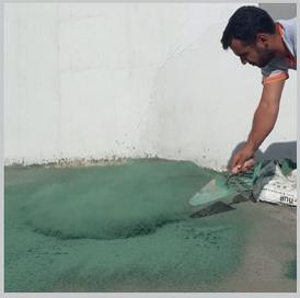
25 kg C-FLOOR-HARDENER surface hardener is ready for use, it is applied as powder. No mortar preparation is required. C-FLOOR-HARDENER surface hardener is sprinkled uniformly and evenly on the entire concrete surface as 5 kg/m<sup>2</sup> for grey color and as 8 kg/m<sup>2</sup> for other colors.
