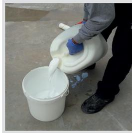
CURE-AR is ready to use, should be shaken before use. If it will be applied with roller, it is poured into a clean and wide bucket.
