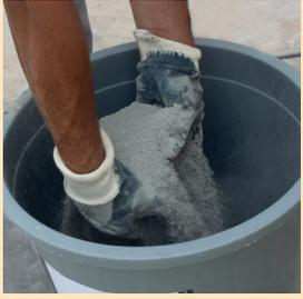
25 kg G-PLAST-MANTO thermal insulation board plaster is added on 6 liters of clean water by sprinkling.
