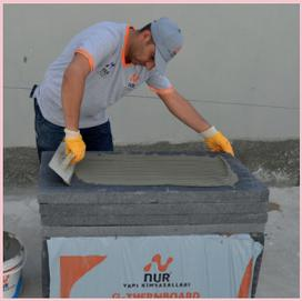
G-FIX-MANTO mortar is applied uniformly to entire backside surface of the thermal insulation board by leaving 5 mm from the edges of board with circular motions using minimum 10 mm notched trowel. Mortar shouldn't overflow from edges of the plate during applicaiton. To get high adhesion strength for fixing of large size-heavy boards, G-FIX-MANTO mortar should be applied both on backside of boards and on to the application surface. Double-sided adhesion should be done.
