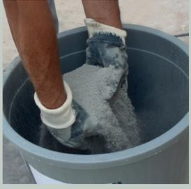
25 kg G-FIX-EXTRA tile adhesive is added on 6,5 liters of clean water by sprinkling.
