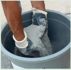
35 kg G-PLAST-1200 hand plaster is added on 7,5 liters of clean water by sprinkling.
