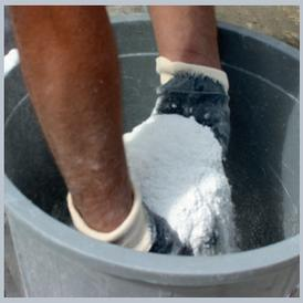
35 kg W-PLAST-POWER fine hand plaster is added on 8 liters of clean water by sprinkling.
